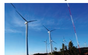
Wind Farm Monitoring (SCADA)
