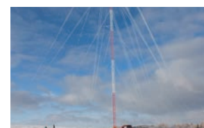
Site Assessment in Cold Climate
